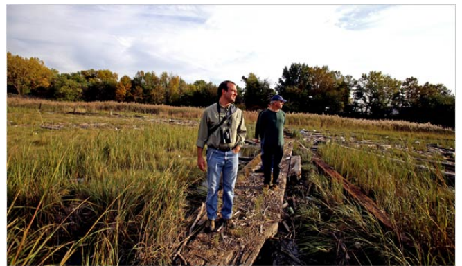
Old planks of decay-resistant hemlock & cedar were all that was needed for this trail across a marsh in Virginia.
